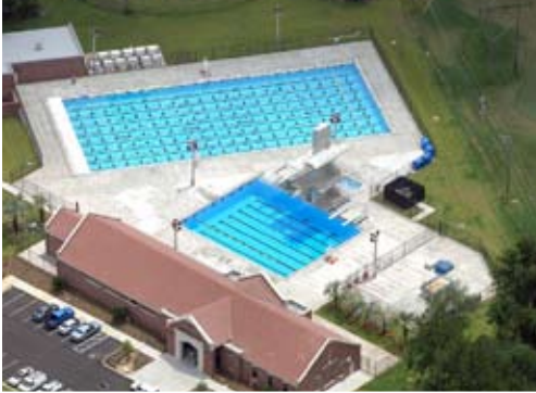
FSU Marine Science Research & Training Facility / Tallahassee, FL.
